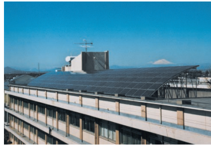
The PV-MY075A roofing material-type photovoltaic battery module blends in with surrounding roofing material so that the modules can go undetected on the roofs where they are mounted. With module miniaturization and the freedom provided by a versatile positioning method, a 4.20kW system can be mounted on a roof that could previously only support a 3.02kW system. Installation time has been shortened through the use of a mounting method in which a stand is not required.
