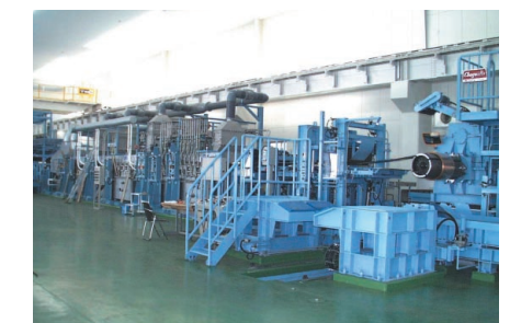
New equipment to remove rolling mill oil
