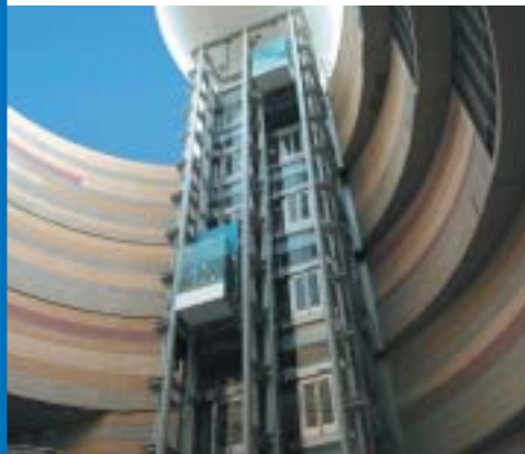
Outdoor-type panorama view elevator for Nanba Parks Building, Osaka Securing an open and unenclosed elevator tower achieves unity with the sound, light and images emerging from the building itself. This development has attracted attention as a "charismatic elevator."
