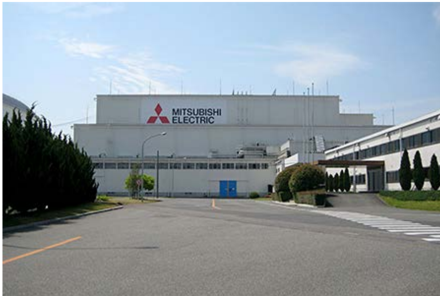
Grid power system factory, Ako Works
