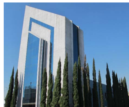
The Mexico City FA Center, located in Mexico Branch of Mitsubishi Electric Automation, Inc.
