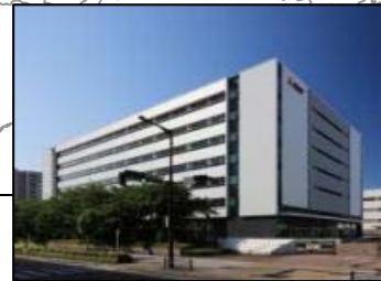
FA Development Center No.2 completed (July 2017)
