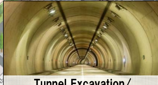
Tunnel Excavation/ Ventilation
