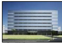
Advanced Technology R&D Center (Amagasaki City)
