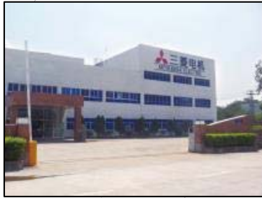
Mitsubishi Electric Low-Voltage Equipment (Xiamen) Co., Ltd.
