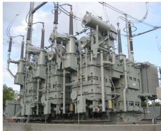
Special divided three-phase transformer
